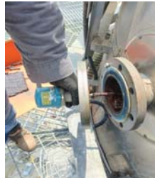
Check and clean temperature sensor unit 2
