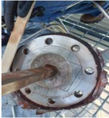
Check and clean probe pressure unit 1
