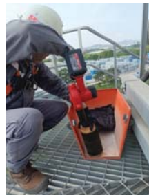
Clean filter blower dust unit 1 & 2
