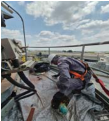
Check and clean temperature sensor unit
