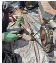
Check and clean probe pressure unit 2
